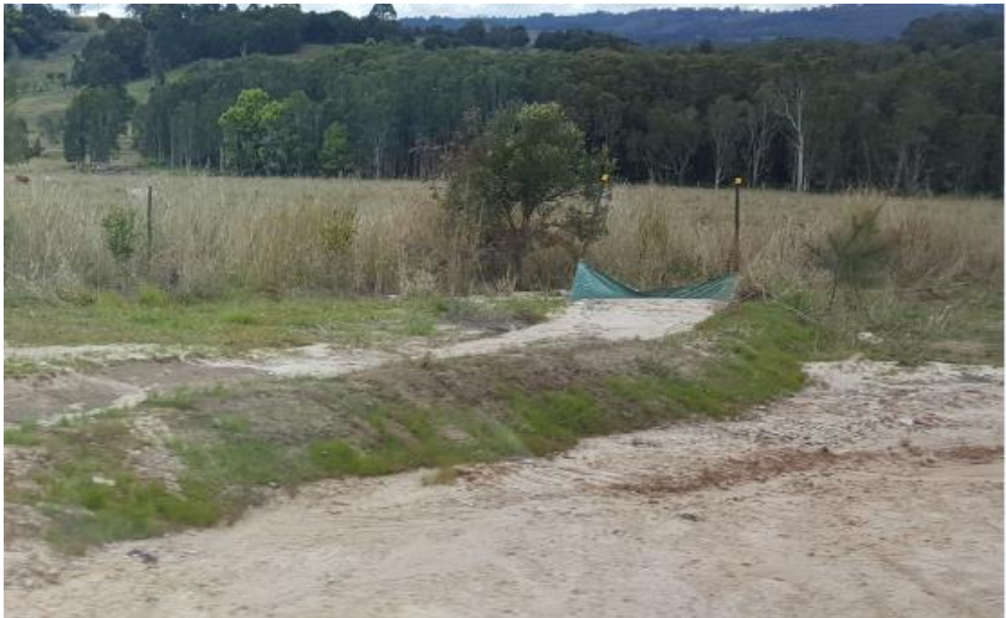
Figure 3-6 Sediment control requiring maintenance
